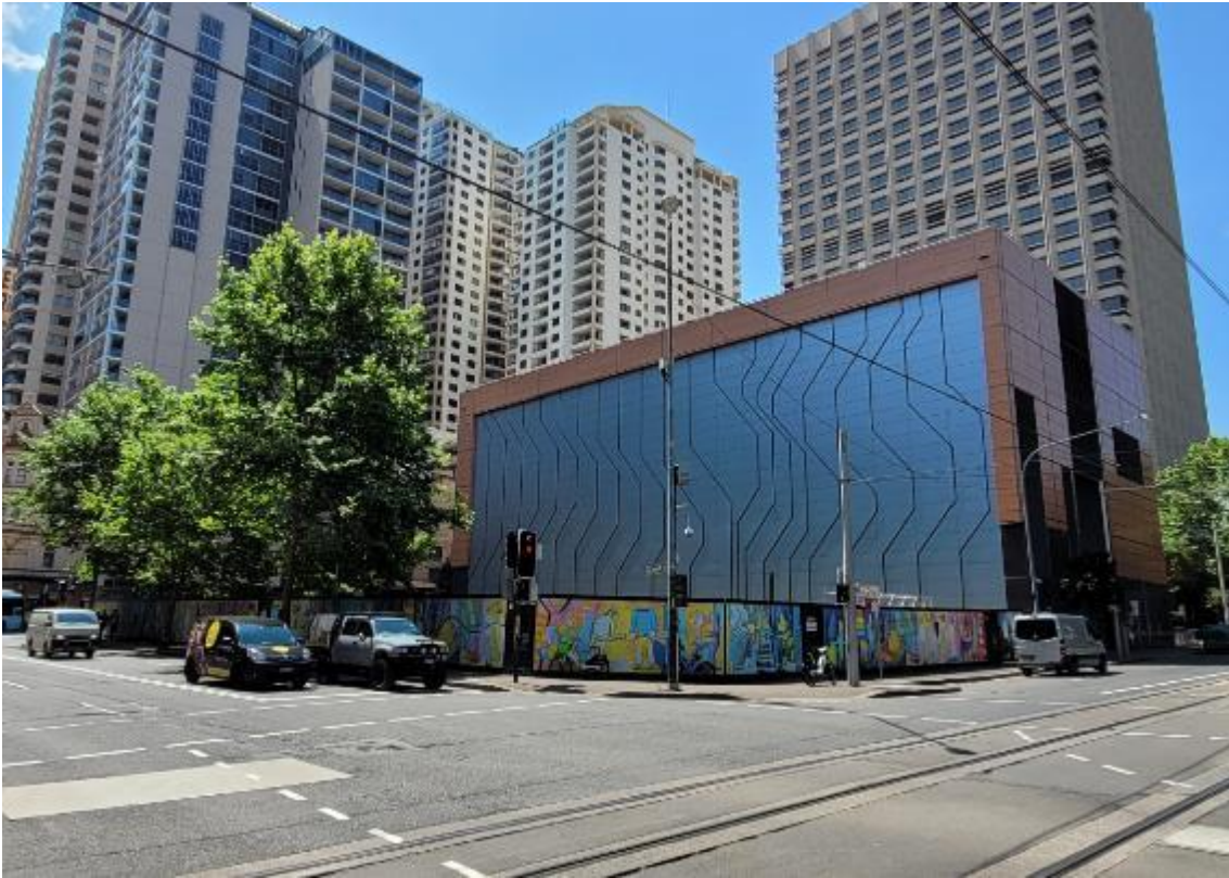
Figure 5: Site viewed from the corner of Hay Street and Pitt Street (generally looking in a north east direction)
