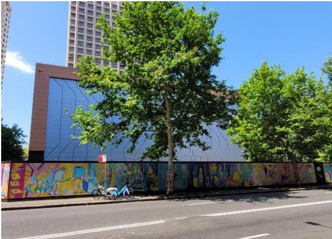
Figure 4: Site viewed from Pitt Street, with the Belmore Park Zone Substation in the background
