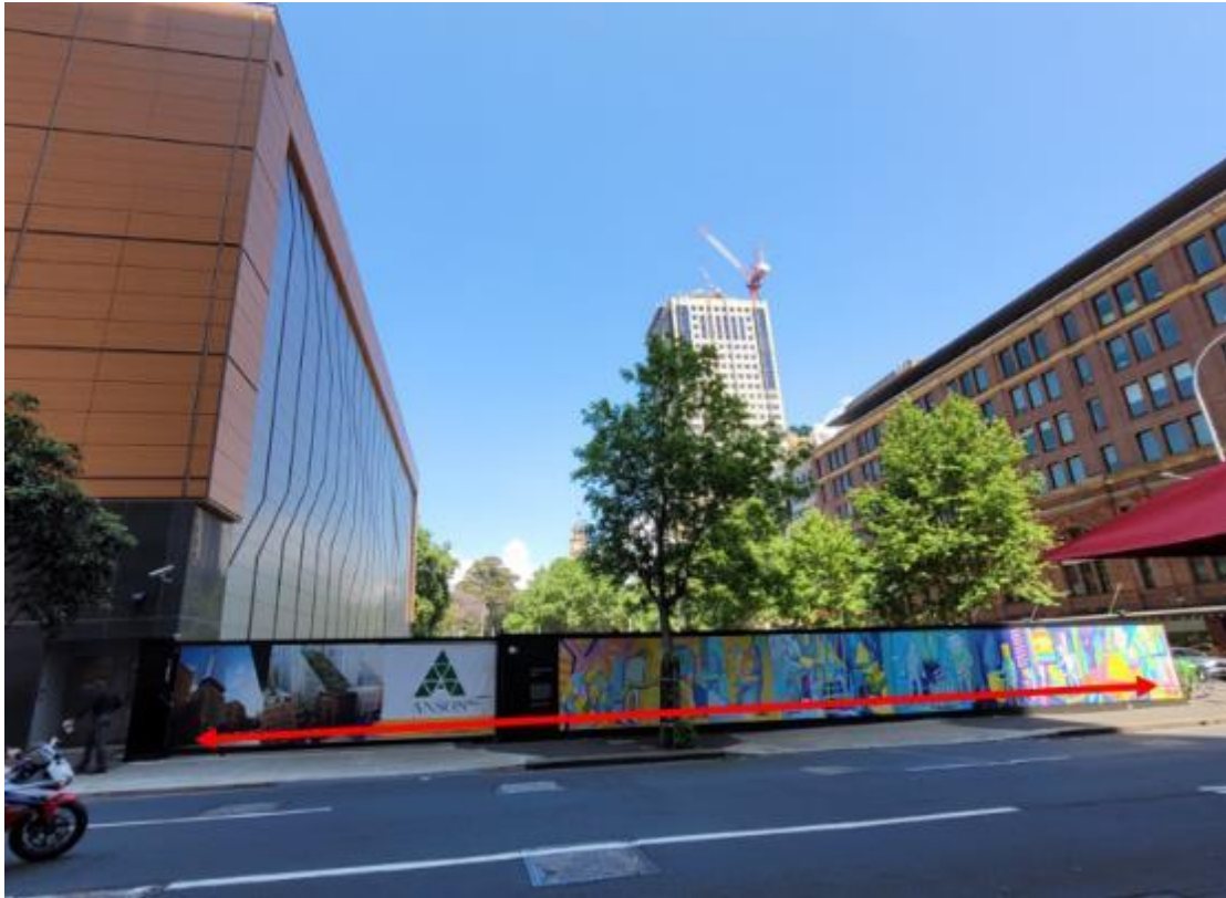
Figure 3: Site viewed from Campbell Street, with the neighbouring Belmore Park Zone Substation to the left
